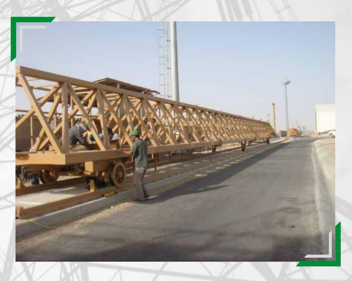
**Scope:** 3 set electrically driven sliding doors located on the Taxiway connecting to Aircraft Parking Area for the security purposes with each has 2 wings each 41 m. and 44 m. long. Project electrical engineering, electrical-mechanical installation,
